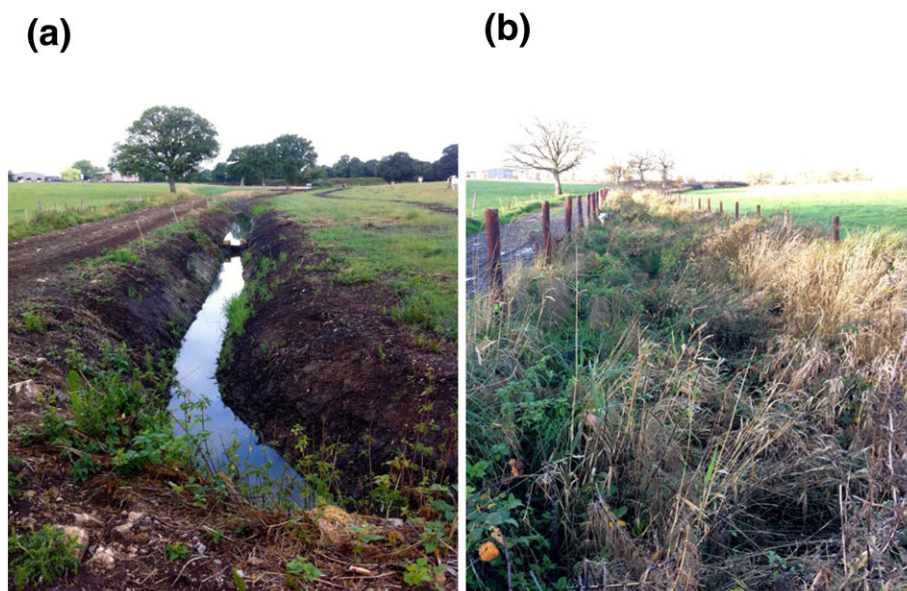
FIGURE 6 View of the drainage ditch on Hays Farm looking from the River Sem to upper farm scale: (a) Post-dredging in July 2013 and (b) dense vegetation and fencing in December 2015 [Colour figure can be viewed at wileyonlinelibrary.com ]
