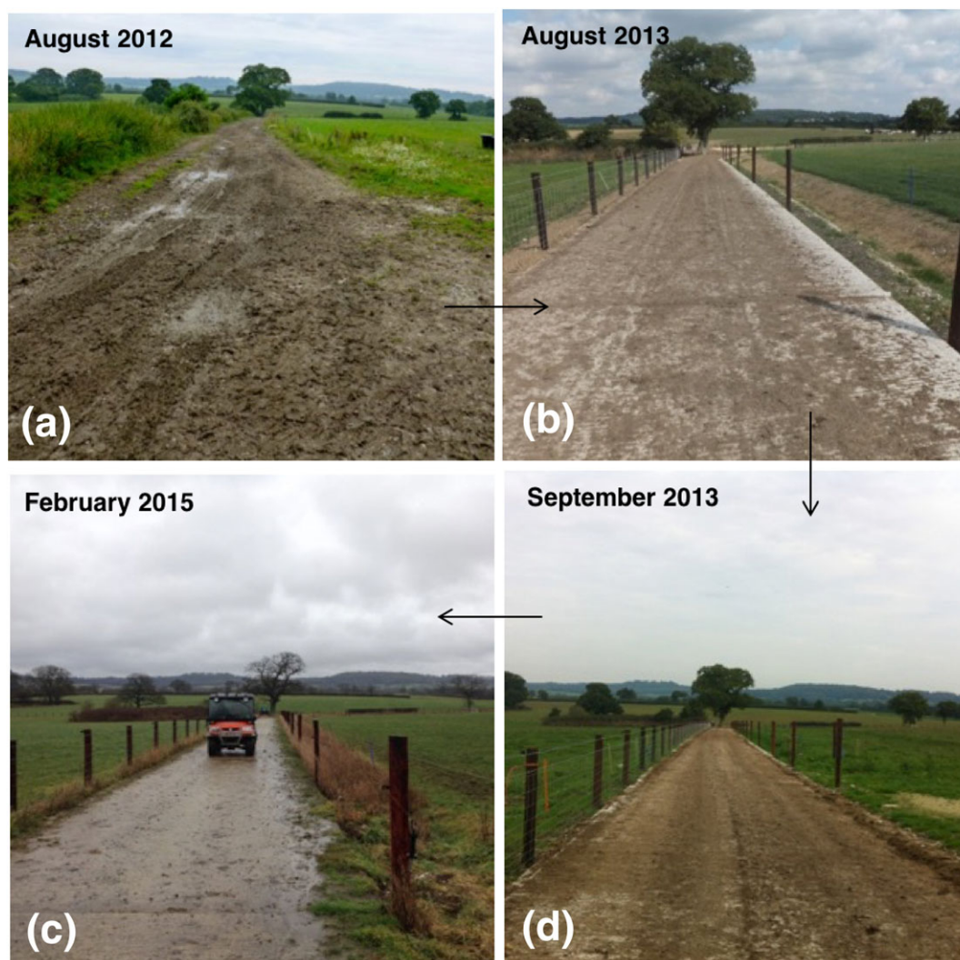
FIGURE 4 Photographs of the upper farm track at Hays Farm. (a) Standing from the farmyard looking downslope pre-mitigation and (b–d) post-mitigation [Colour figure can be viewed at wileyonlinelibrary.com ]
