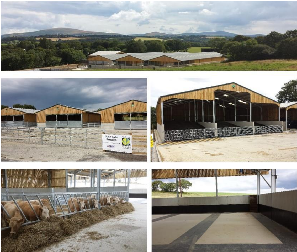
Figure 14. Dedicated cattle housing, silage clamps and FYM middens at North Wyke, Rowden site.
