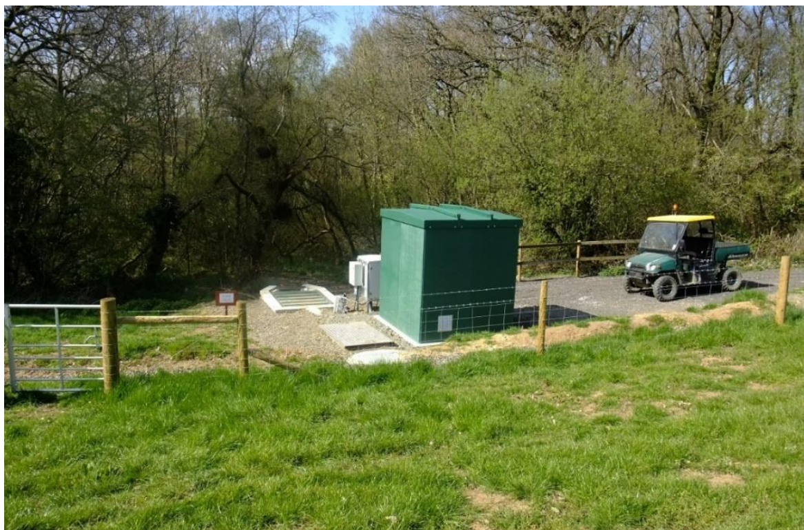
Figure 16. One of fifteen flume cabins which are sited at each catchment.
