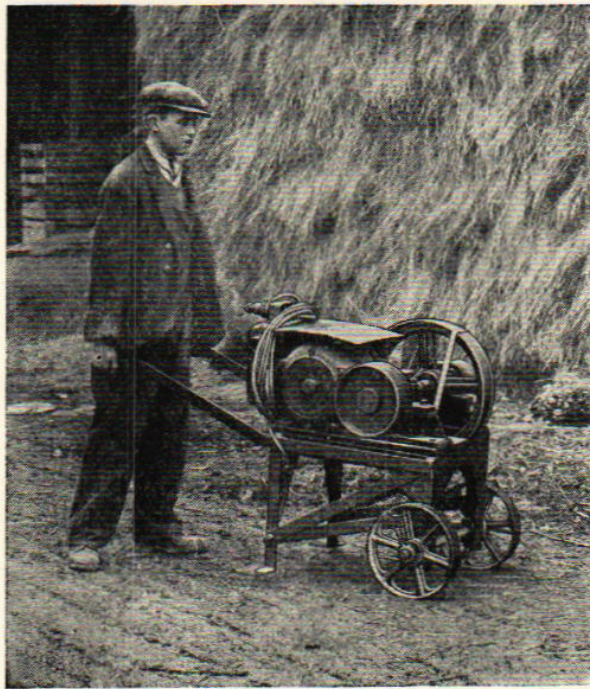
Fig. 9. 5 h.p. portable motor and countershaft on two-wheeled truck, to 7\frac{1}{2} h.p., whilst over this size, due to the greater weight, four-wheeled construction is preferable. Although the majority of designs are a combination of trucks on which the motor and control gear are mounted, there is one notable exception, namely the
