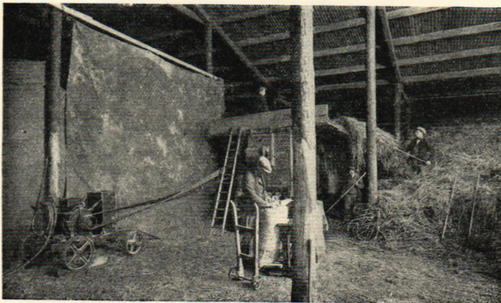
Fig. 11. 20 h.p. heavy duty portable motor driving thresher.
