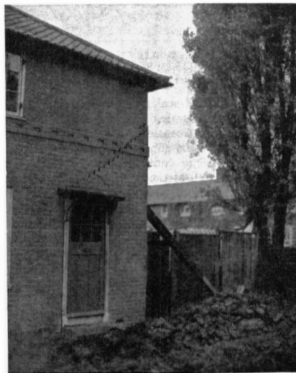
Fig. 7. Damage to a house, caused by shrinkage of clay soil, Edgware, 1947 [Crown Copyright reserved]
